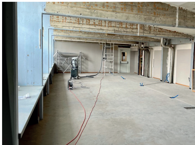
Library under renovation
